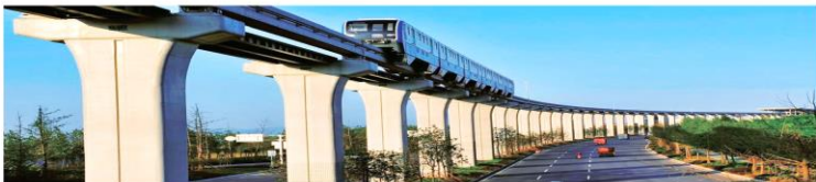
The first straddle monorail in China - Jiaochangkou-Xinshancun line in Chongqing was awarded Top 10 Construction Technology Achievements in China.
