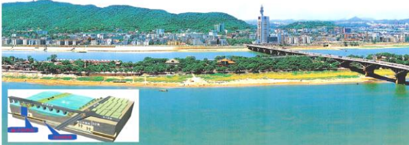
长沙2号线穿越湘江工程——我国地铁工程设计穿越大江大河的最具代表性的项目，解决了诸多国内罕见难题 Changsha Metro Line 2 crossing Xiangjiang River – the most typical project of metro line crossing large river in China, which solved many rare technology challenges
