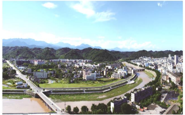
法国贷款大邑市政基础设施灾后重建项目，采用EPC总承包模式，在国内灾后建设和利用外资领域的属首次。 Post-Disaster Construction Project of Deyang Municipal Infrastructure with French Loan is executed under the mode of EPC Contract, which is the first for post-disaster reconstruction project using foreign loans.
